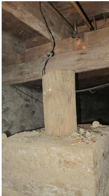
Figure 25 Reused Beam
