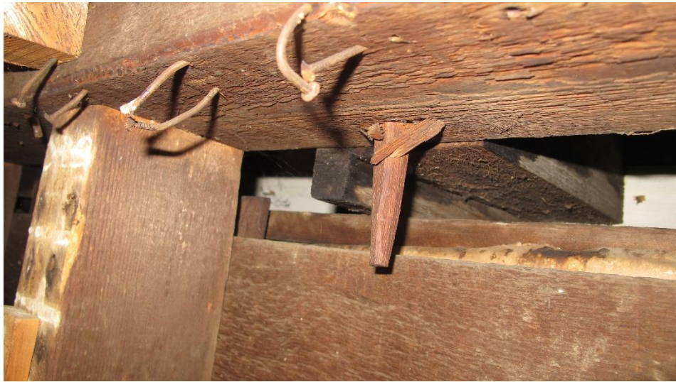
Figure 22 2017 peg mortise and tenon joint at boxed eave
