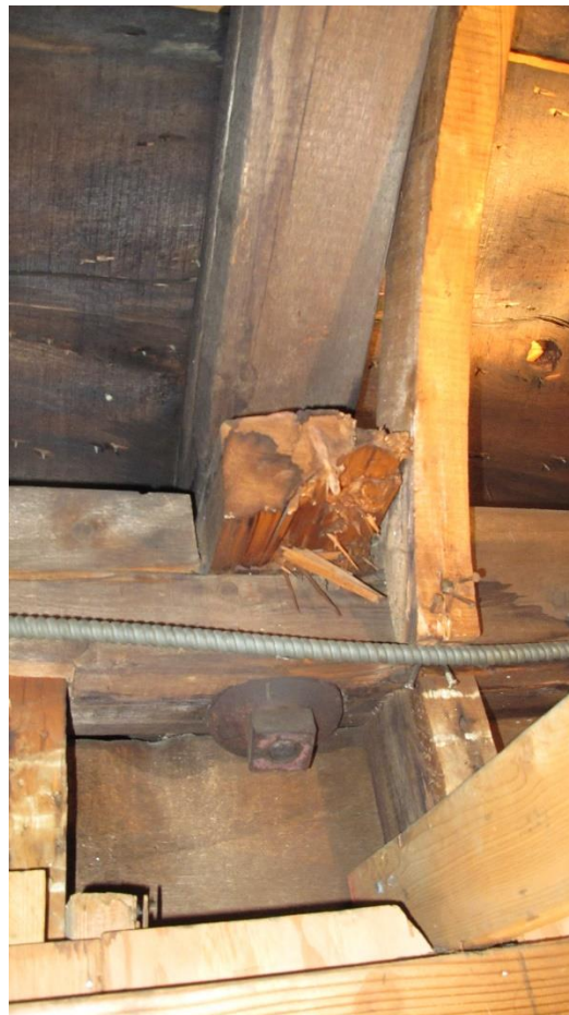
Figure 23 Heavy timber of early Greek Revival structure with iron bolt
