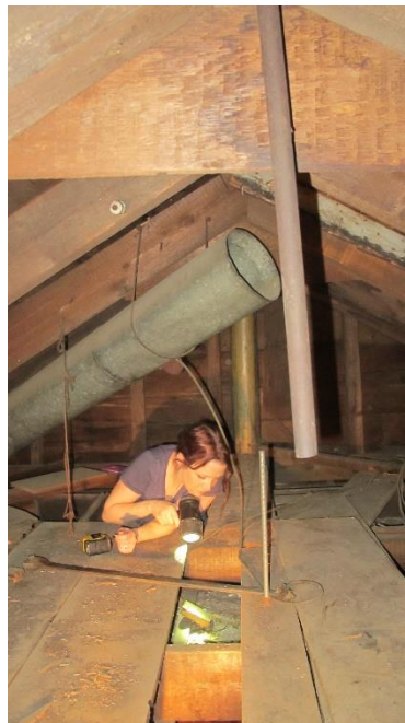
Figure 7 Roof peak, iron sag rod in foreground, projector vent pipe visible, flag pole remnants at rear center
