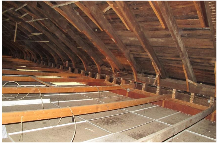
Figure 6 Interior vaulted roof structure above drop ceiling, main hall
