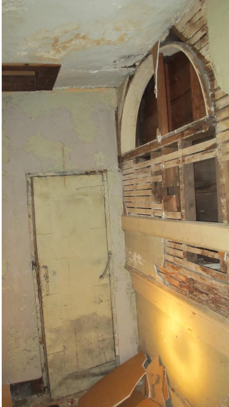
Figure 11 Taken on balcony, metal projector room door visible, street side fan window visible at top right also boarded up on exterior (SHPC 2017)
