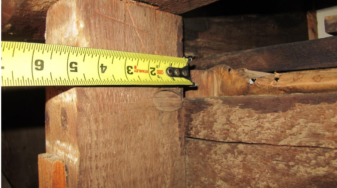
Figure 27 Mortised wall stud to eave girt
