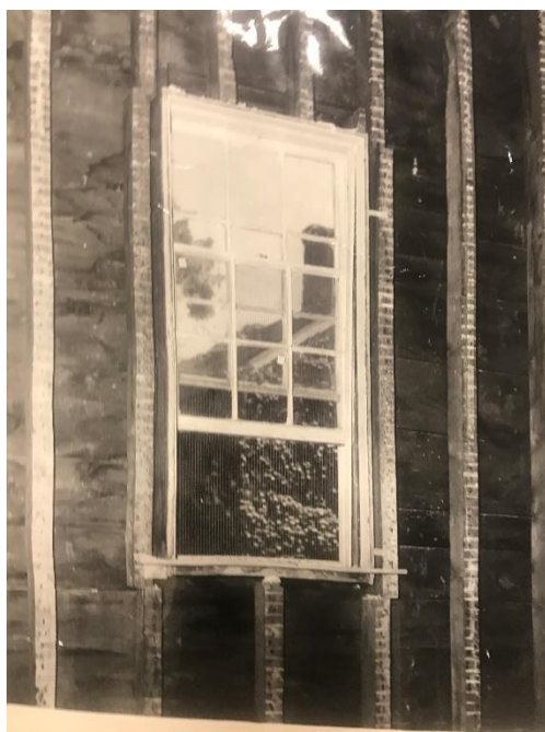
Figure 21 9 over 6 sash c.1906 (this photo is not current condition, photo taken 1954)
