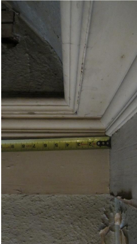
Figure 8 Mouldings under arch ceiling soffit at ends
