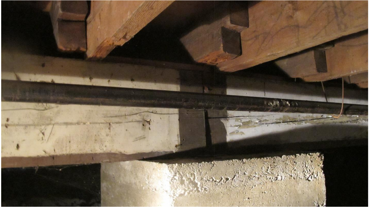
Figure 24 (above) Reused joists
